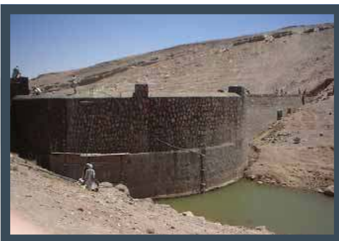
Illustration 13: Dam under construction
