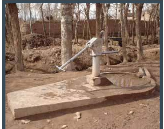
Illustration 16: Well handpump (Bob Rout photograph)
