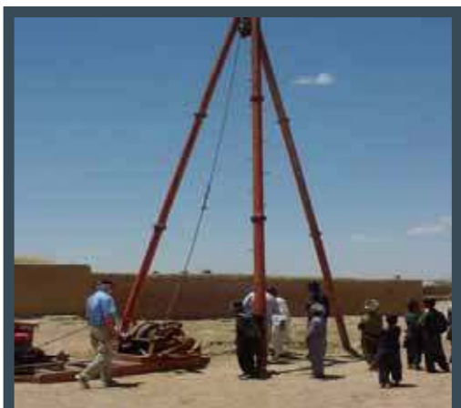
Illustration 19: Modern well-drilling (Bob Rout photograph)
