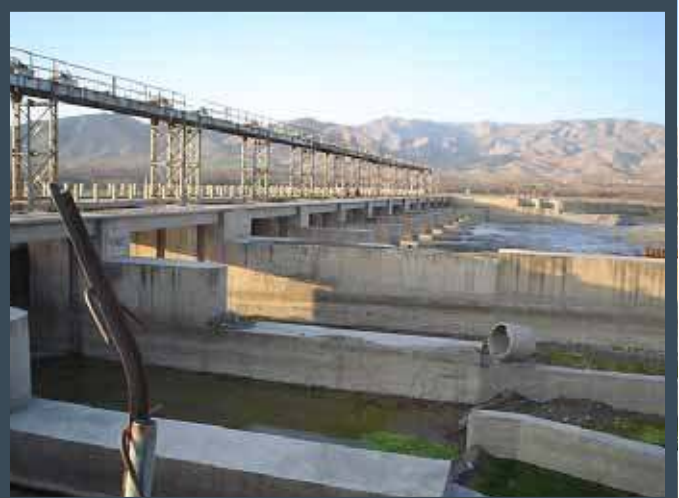
Illustration 21: Diversion weir, Kunduz-Khanabad (Bob Rout photograph)
