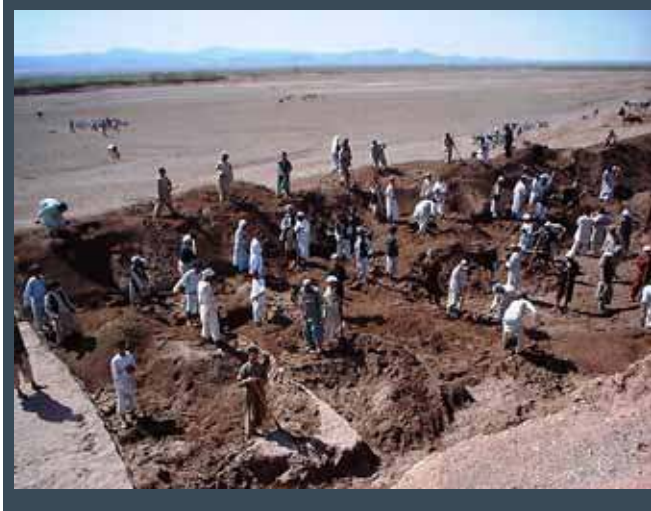
Illustration 1: Annual maintenance on Joy Naw main canal, Herat (Bob Rout photograph)
