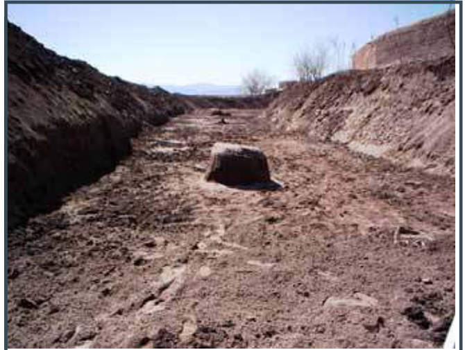
Illustration 3: Main canal after de-silting
